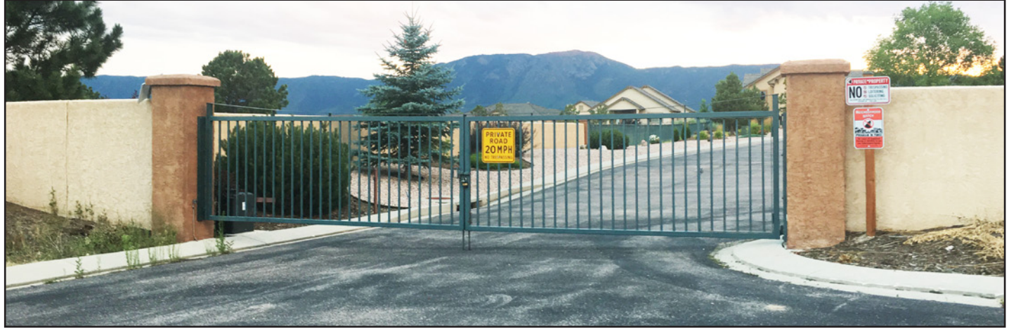
Above: Brookmoor Estates has requested a Planned Use Development amendment from the county to allow residents to use this gate at the back of the development to access South Park Road. The county project manager is Kari Parsons (kparsons@elpasoco.com). See www.ocn.me/v12n10.htm#brookmoor . Photo by Jackie Burhans.
