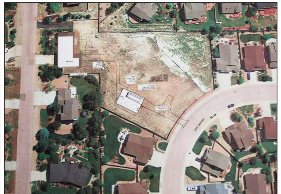
Above: The proposed site along Homeland Court for Donala Water and Sanitation District's Water Treatment Plant Residuals Dewatering Facility. The structure will house a plate filter press to "dewater" liquid waste into disposable solids directed to municipal landfill instead of the Upper Monument Creek Regional Wastewater Treatment Facility, which faces more restrictive biosolids regulations as of Oct. 1. Photo by Jennifer Kaylor of the graphic presented at the meeting.
