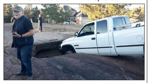
**Above:** A broken watermain caused a sinkhole that ate a truck on Caribou Drive West in Woodmoor and affected traffic on Oct. 22. The front of the truck got stuck in the water-filled hole. The watermain break affected 25 to 30 homes in South Woodmoor Preserve. It was fixed by the Woodmoor Water and Sanitation Department. *Photo by Scott Henderson*.
