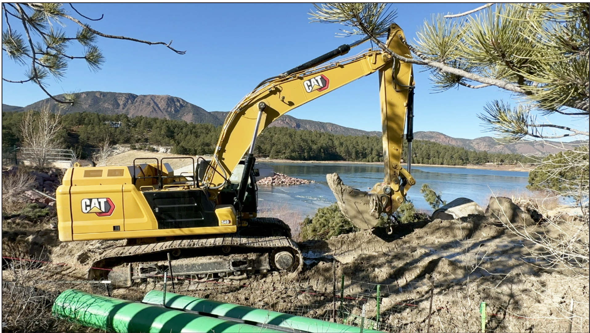
Above: Monument Lake closed on Dec. 5 for a sewer improvement project. Palmer Lake Sanitation District is upgrading the main sewer line from 12 inches
