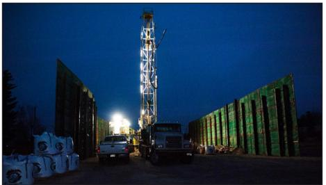
Above: Monument's Well 13 near Santa Fe Trail and Fourth Street had a drilling rig operating 24 hours a day with a sound barrier wall and a well-lit tower and work space. The drilling took place over the last few weeks and is now completed, providing water for Monument's residents. Photo by Jackie Burhans.
