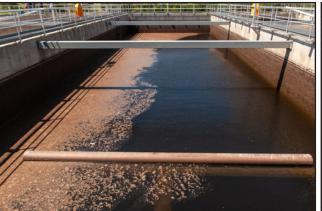
treatment facility operations, and Plant Operator Aaron Tolman led a tour of the facilities, including the three sequencing batch reactor basins. From left, the first basin is aerated by blowers to provide oxygen for the microorganisms that process the
