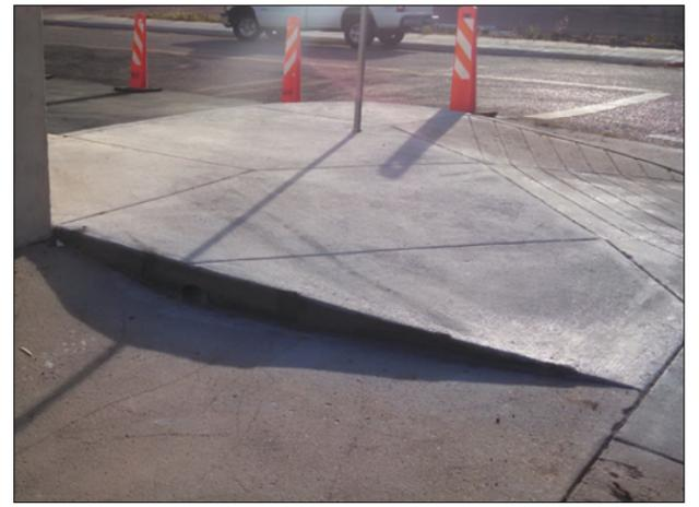
**Above:** The town's new sidewalk along the west side of the Monument Sanitation District building has created a tripping and icing hazard in front of the entrance to the 2nd Street Hair Salon. The town has declined to remove the problem portion of the new sidewalk and reinstall replacement concrete at the correct grade to eliminate the hazard as requested by the district. Photo by Mike Wicklund.
